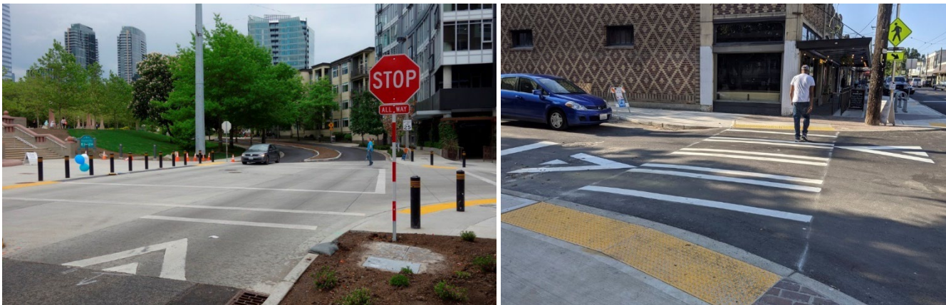
Figure 20: Example of Raised Crosswalk and Raised Intersection
