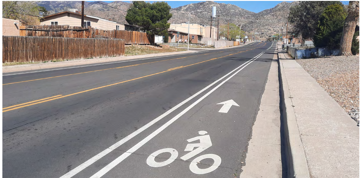
The travel lanes on this section of Copper Avenue east of Chelwood Park Boulevard were recently narrowed to create space for a striped buffer.
