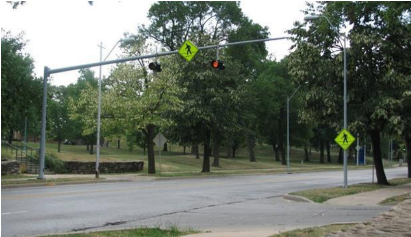
Figure 14: Overhead Flashing Lights Example
