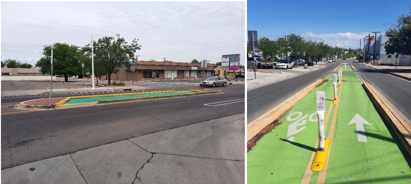
Figure 15: Examples of Staggered Crossings with Raised Medians along Bike Boulevards in Albuquerque
