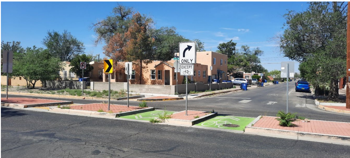
Figure 22: Raised Median along Silver Ave Bike Boulevard
