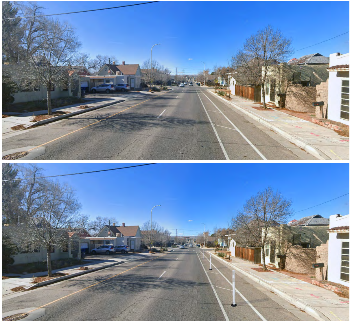
Figure 18. Existing Buffered Bike Lanes (Top) and Option for Separated Bike Lanes (Bottom)
