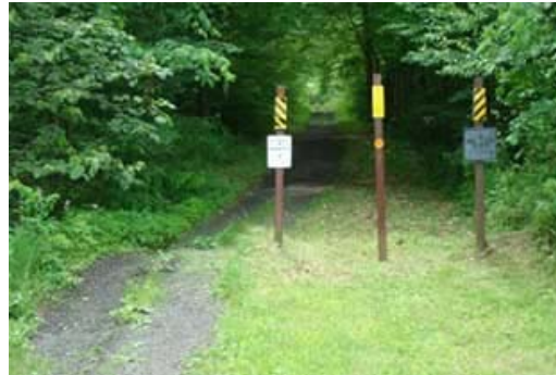
Photo of bollards on the Delaware and Hudson Rail Trail in Pawlet VT. Trail users created a new trail to get around the bollards. Photo by Jon Kaplan, Bicycle and Pedestrian Program Manager, Vermont Agency of Transportation.
